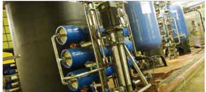
Kraft Foods' new membrane plant treats water for reuse in cooling towers
