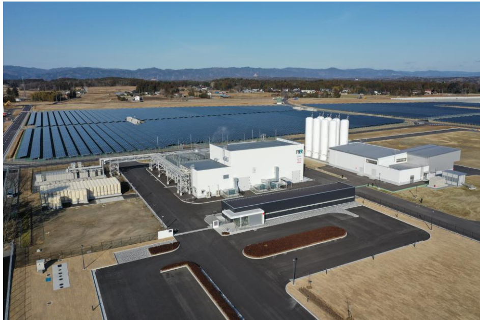
Solar to Hydrogen Electrolyser in Fukushima
